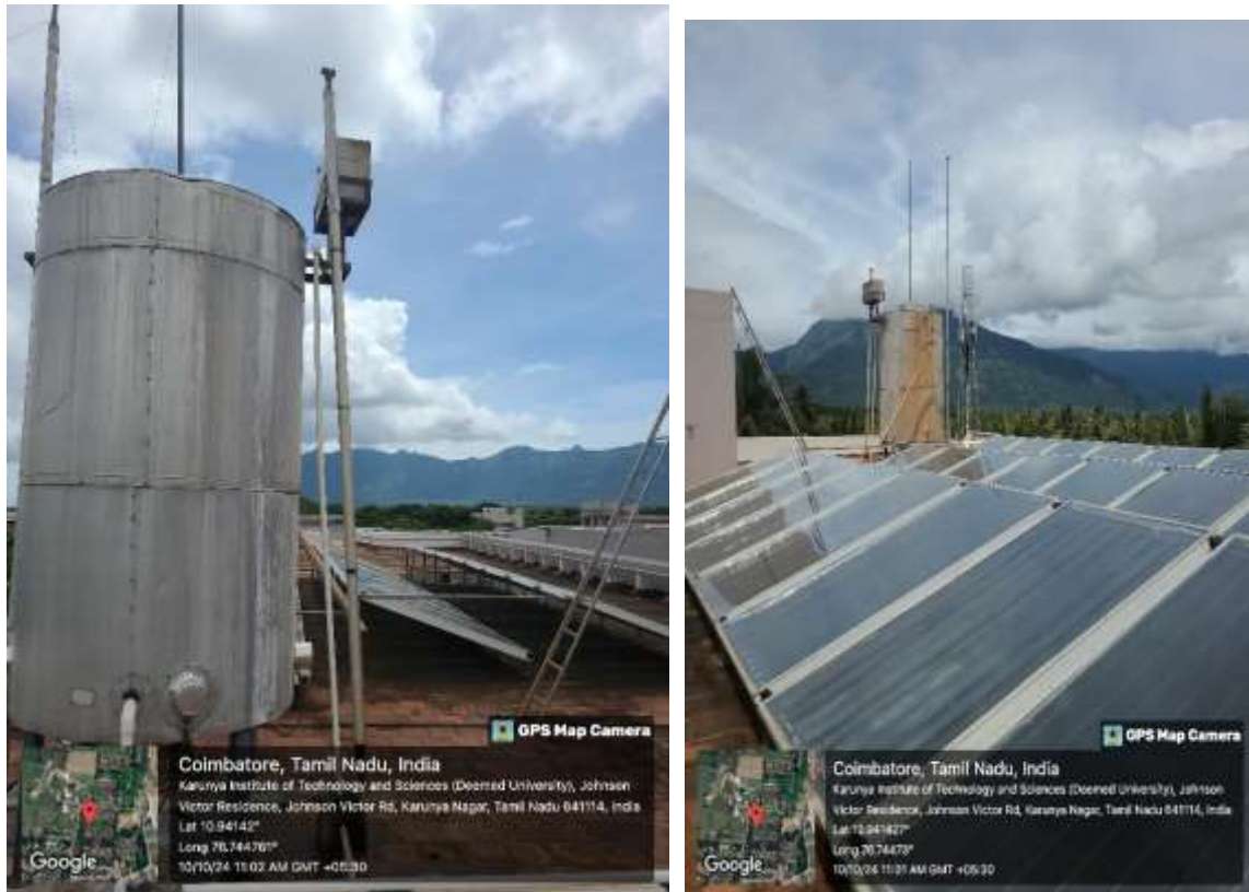
Fig 7. 87,600 LPD Solar Water heating system (30 Nos): 15,45,718 kWh
