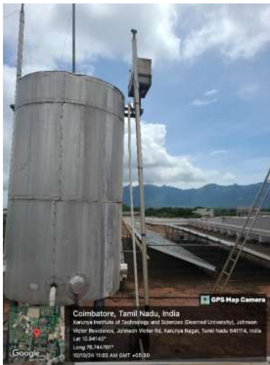
87,600 LPD Solar Water heating system (30 Nos): 15,45,718 kWh
