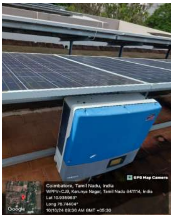
Fig 5.95kW Solar Power Plant in Admin Block: 87,473.71 kWh
