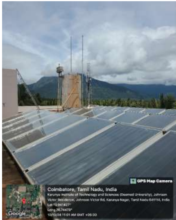
87,600 LPD Solar Water heating system (30 Nos): 15,45,718 kWh
